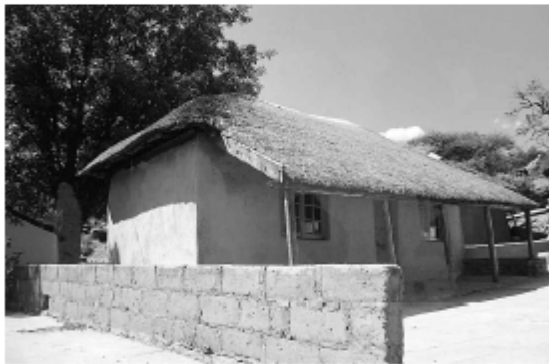
Fig. 4. Sun-dried earth block wall supporting thatched roof.
