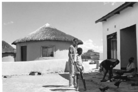
Fig. 1. Mud wall with thatched roof (left); and concrete brick wall supporting corrugated iron sheet roof (right).
