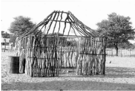
Fig. 2. Vertical poles before in-filling with mud.
