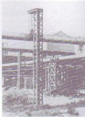
Figure 1: Example of a laced column in mineral industry
